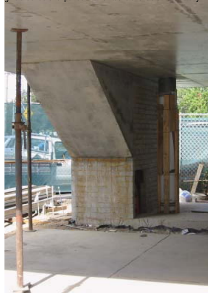
PARK STREET HOUSE - Construction
